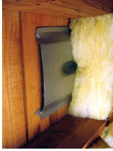
Rafter vent—in gray above—installed between rafters where the roof meets the attic floor.
